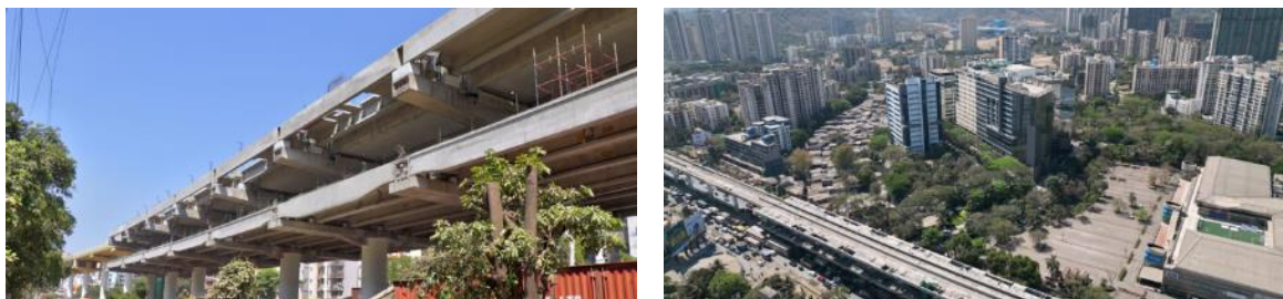
Figure 16: Metro progress outside G Corp Tech Park; Source: JLL Report
