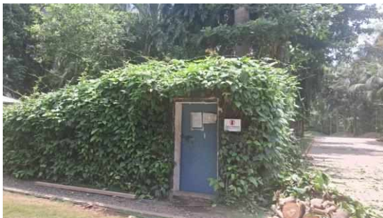
External View of STP in Subject Project
