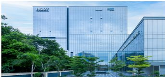
WeWork HQ27, Gurgaon
