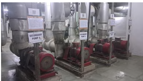
View of Chiller Auxiliary Pumps in Subject Project
