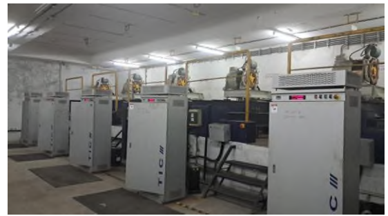
Internal View of Lift Machine Room at Subject Project
