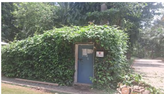
External View of STP in Subject Project
