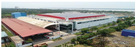
Manufacturing plant: Falta, West Bengal
