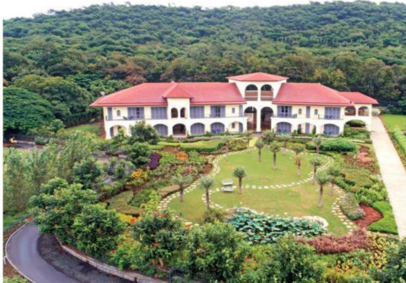
“The Source at Sula” facility in Nashik, Maharashtra
