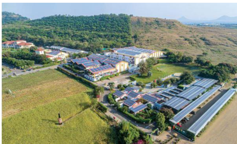
Our facility at Nashik, Maharashtra
