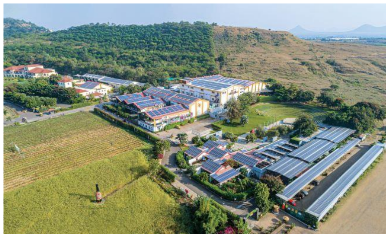
Our facility at Nashik, Maharashtra
