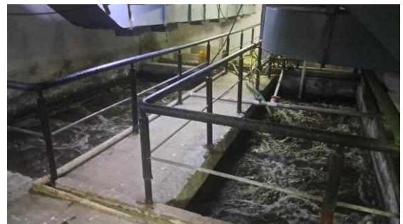
Internal View of STP in operation in Subject Project
